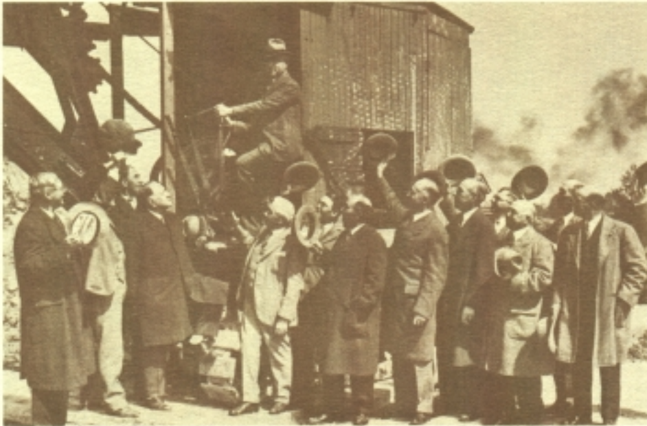
Groundbreaking ceremonies for the plant project were held May 26, 1930, as Port Washington Mayor August F. Kruke manned the steam shovel.
