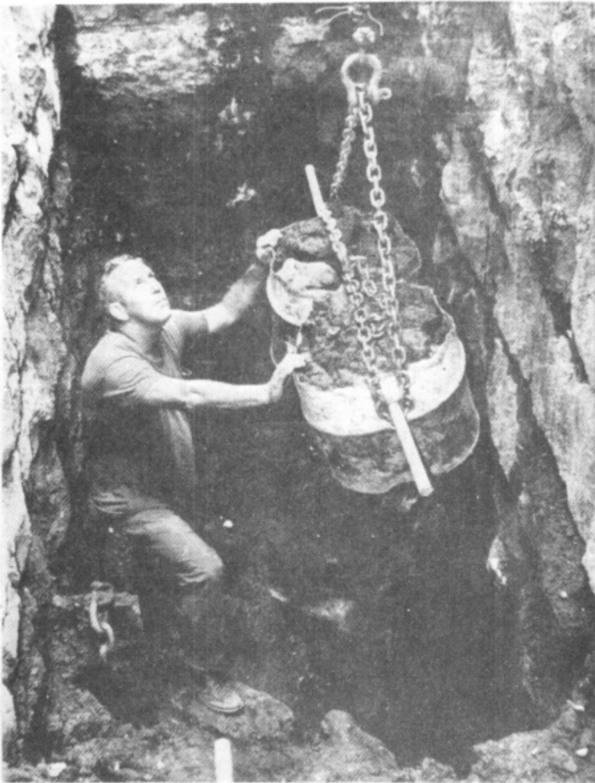
Jim Lee guides a load of debris out of the turbine chamber as the excavation proceeds
