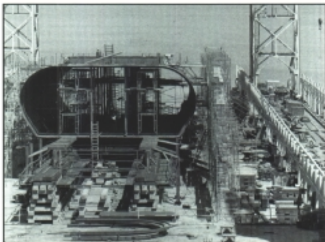
The BART Transbay Tube under construction.
