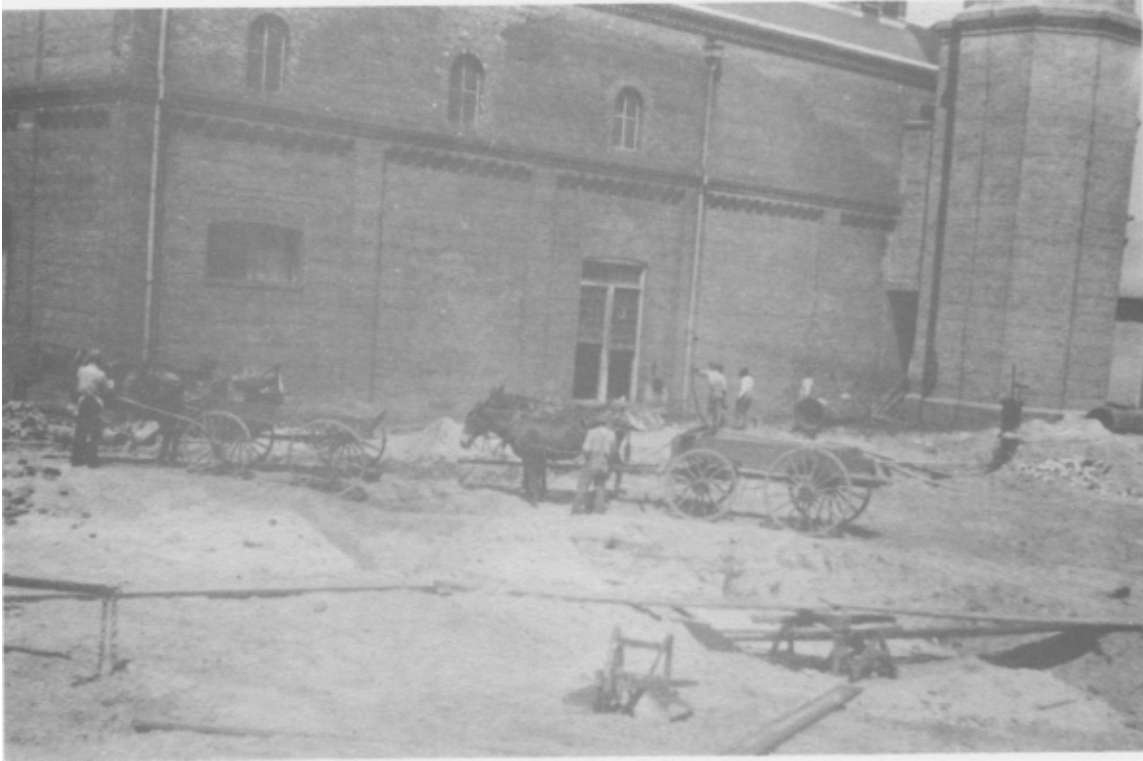
OUTSIDE VIEW OF BOILER ROOM. NEW PUMPING STATION GROUND BEING PREPARED IN 1914.
