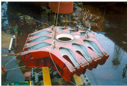
Thordon SXL bearing installed in FPSO turret application
