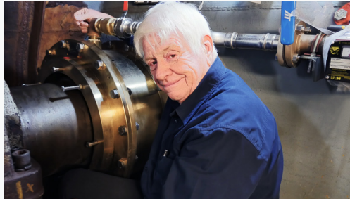
Sandy onboard the Canadian Coast Guard Ship Hudson with SeaThigor mechanical face seal installed.
