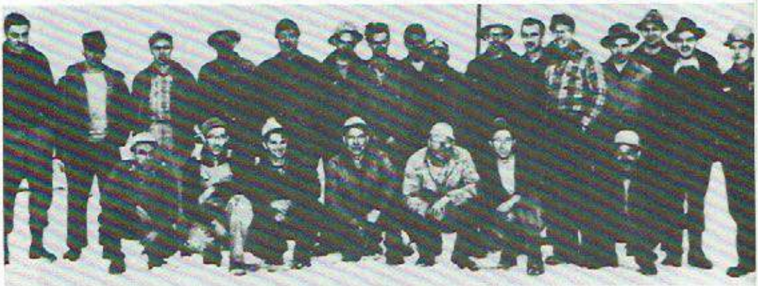
Fig. 11. Consolidation Coal Pipeline Crew - Early ' 50's
